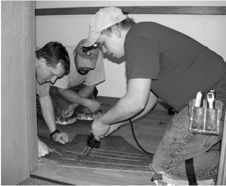
In October, floor covering apprentices used new heat welding kits, arc cutters and other tools purchased through a Wisconsin Sector Alliance for the Green Economy (SAGE) grant to install Teknoflor sheet vinyl throughout the Eastern Training Center
