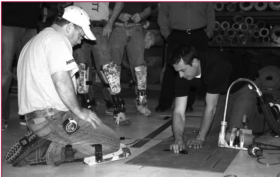
The INSTALL Floor Coverers Training Center in Saint Paul, Minn., hosted Mike LeClair (right) of Protect-All Commercial Flooring to give an upgrade class in how to apply their vinyl flooring. The class was presented in conjunction with Hank's Specialties, a flooring and installation wholesaler. Members learned how to apply the recycled vinyl product, which is perfect for use in areas that get wet such as kitchens, entryways, gym floors and more. Learning to apply specific flooring types and brands gives members a competitive edge. Pictured with LeClair is Tom Wolfe (left), Local 68.
