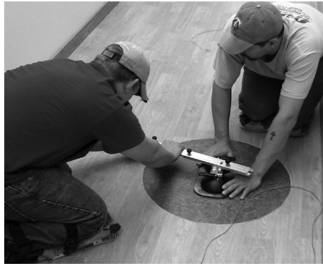
In October, floor covering apprentices used new heat welding kits, arc cutters and other tools purchased through a Wisconsin Sector Alliance for the Green Economy (SAGE) grant to install Teknoflor sheet vinyl throughout the Eastern Training Center
