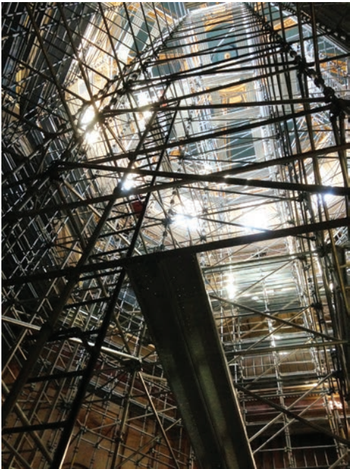
Scaffolding up through the Capitol ceiling dome.
