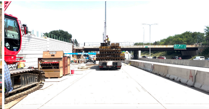
Photo of Blue Line job site in Saint Paul, MN.
